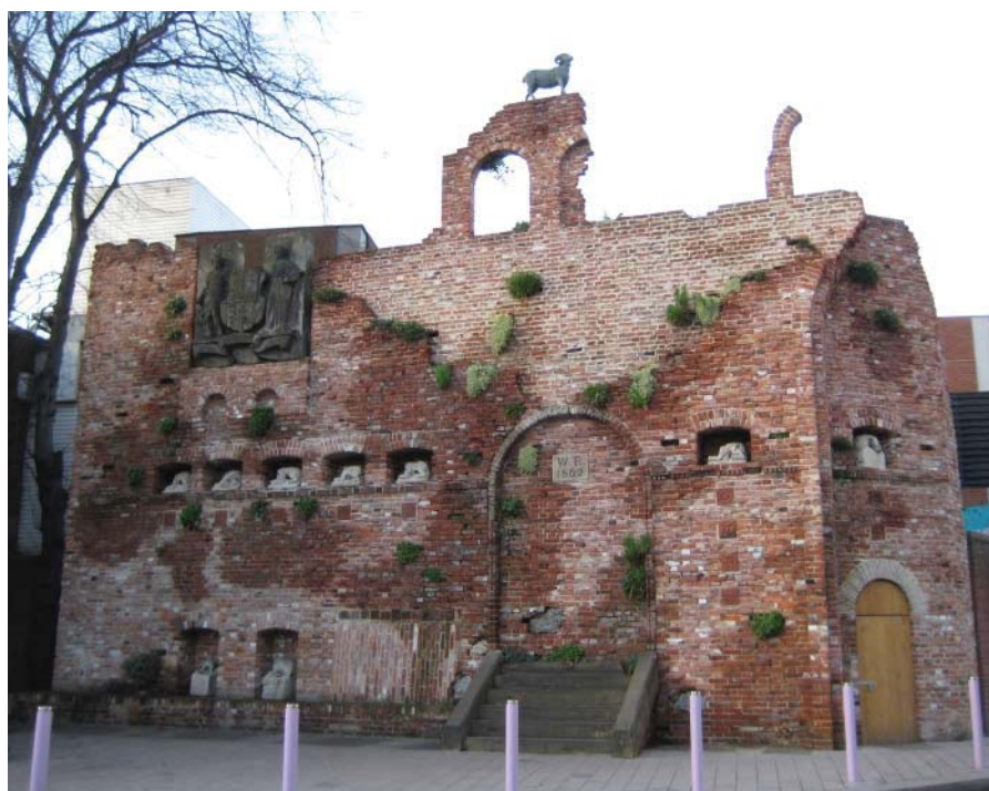
Above Barking Town Square folly by MUF Art Architecture with example of bollard from Barking Town Centre street furniture palette in the foreground
